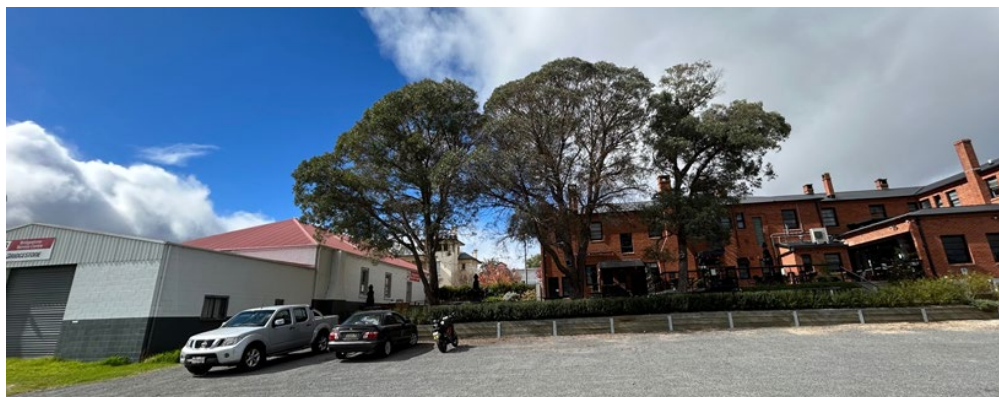
Figure 7 – Western elevation from rear of Commercial Boutique Hotel
