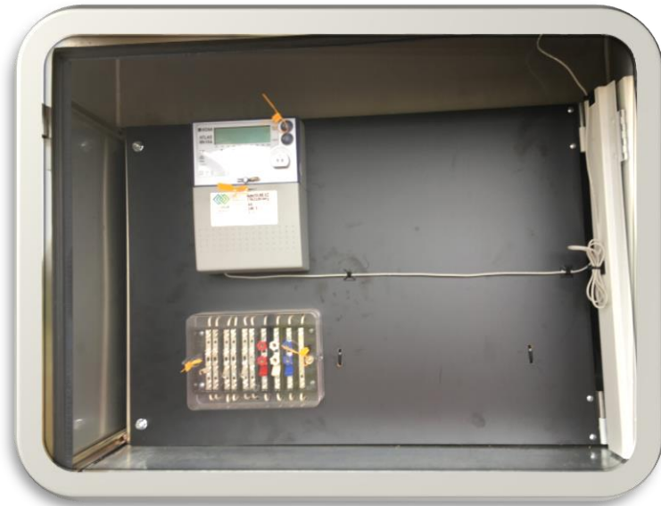
Figure 1 Completed meter installation RFS January 2021
