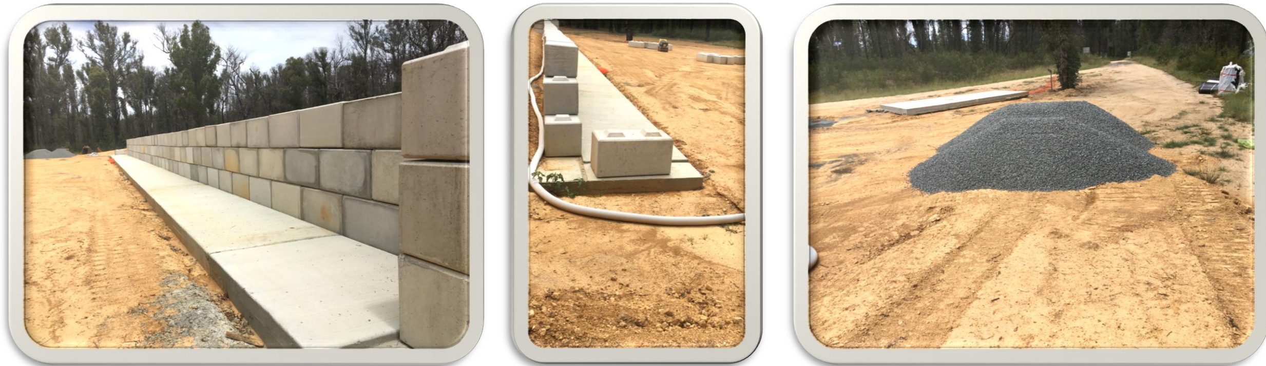
Figure 1, 2 & 3 New Bin Slab and blockwork, drainage line and tip shop slab at Torrington January 2021
