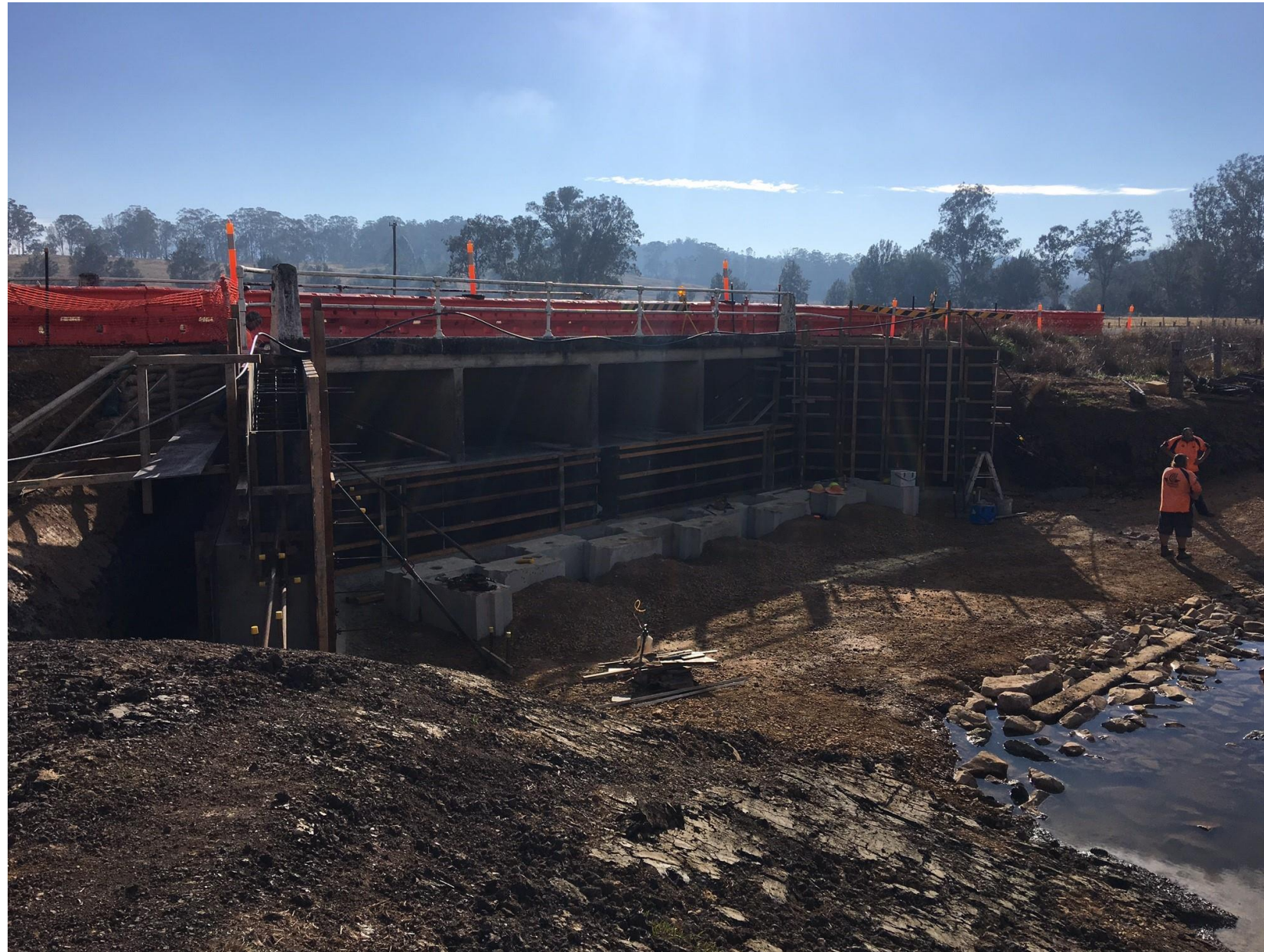
Formwork setup ready for a pour on Woodenbong Culvert
