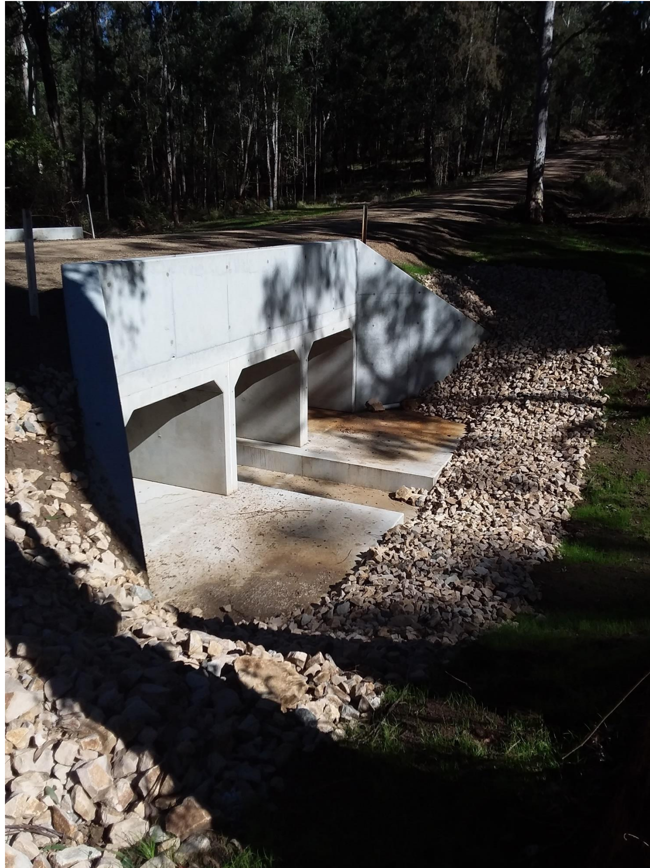
Headgate Culvert
