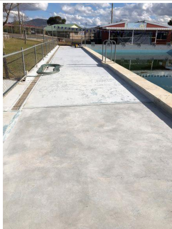
Swimming Pool Concourse – Before (rear) & After (front)
