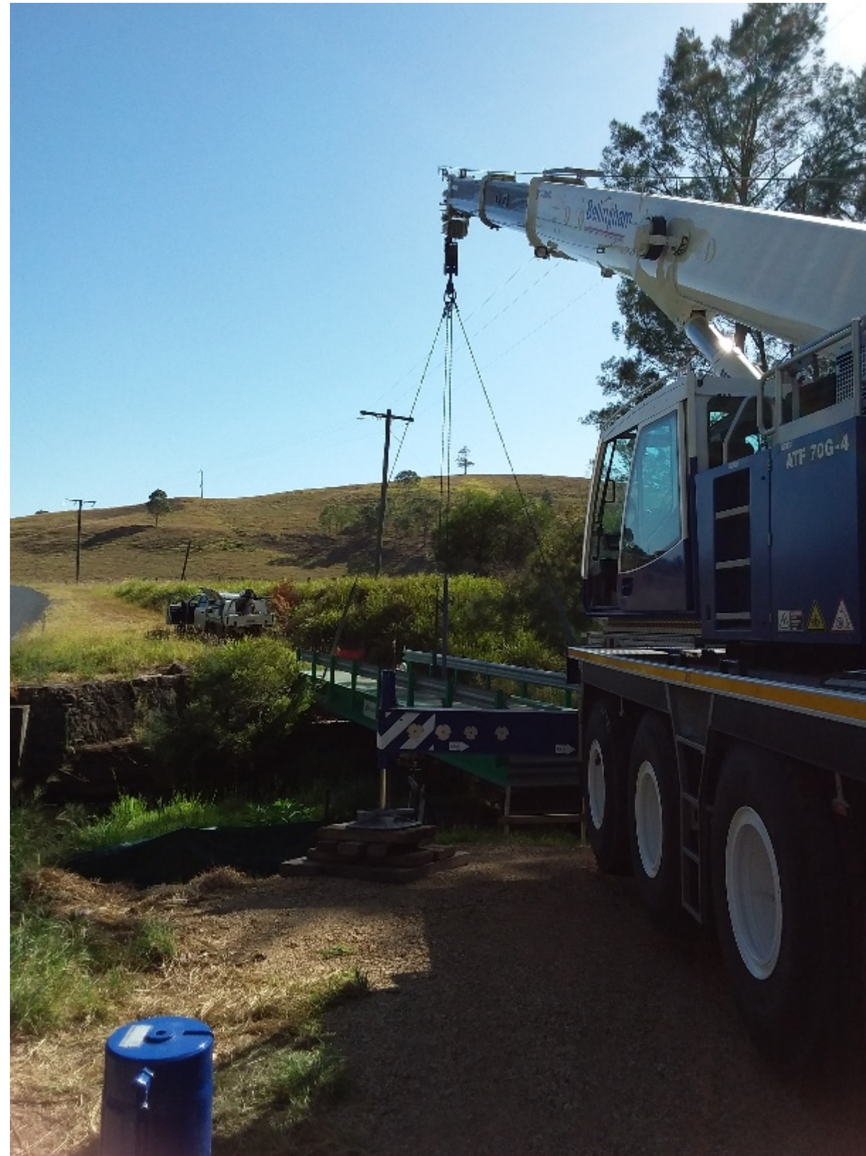
Placing of bridge for Side track on White Swamp.
