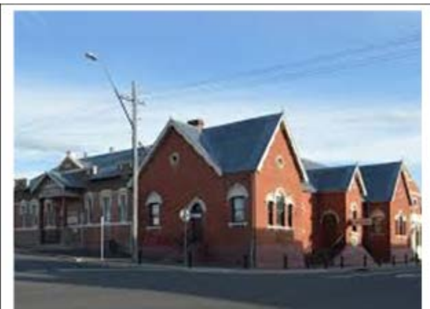
School of Arts Window Restoration Project
