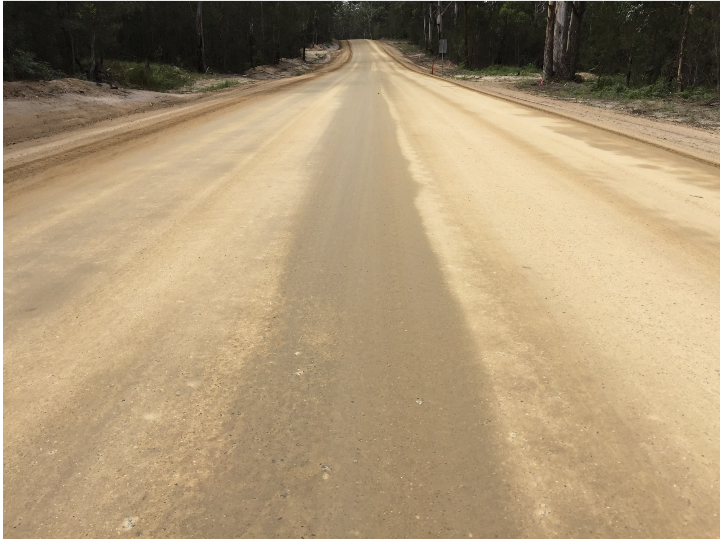
Bald Rock Job – modified pavement
