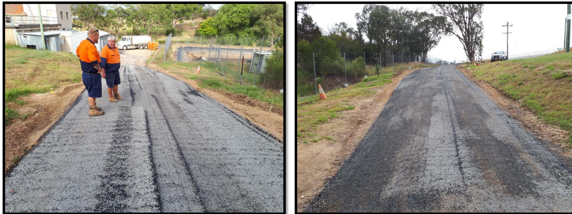
Figure 3 & Figure 4 Tenterfield Water Treatment Plant road seal
