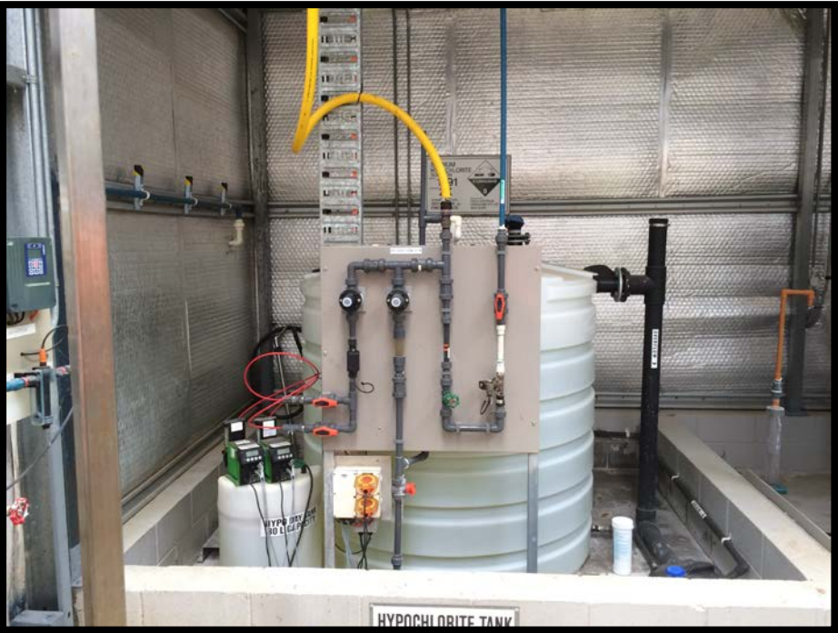
Figure 9 & Figure 10 EPA Urbenville WTP (Water Treatment Plant) chemical dosing
