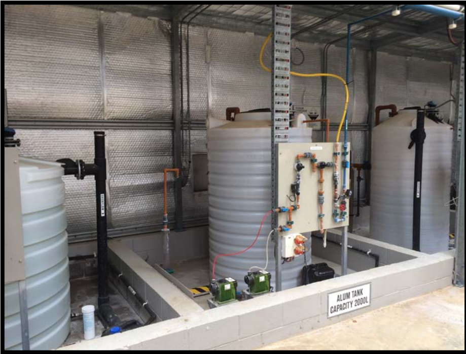
Figure 9 & Figure 10 EPA Urbenville WTP (Water Treatment Plant) chemical dosing
