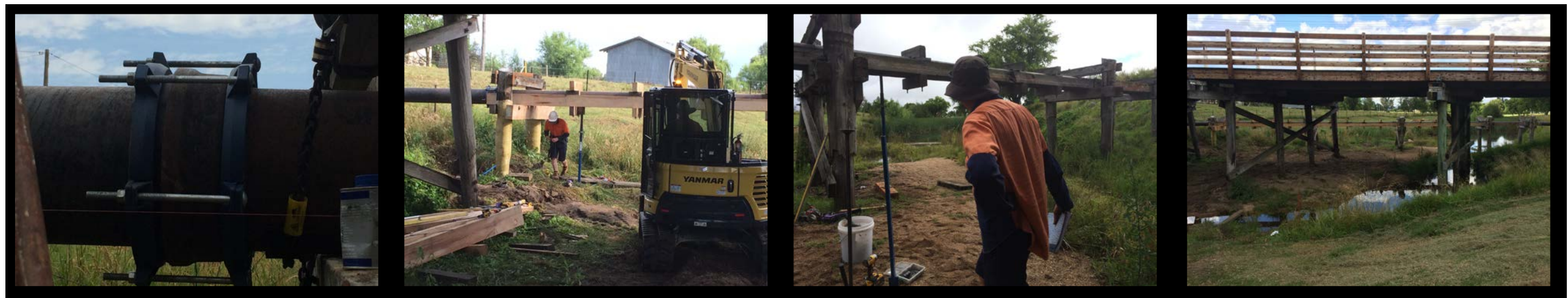
Figure 1, Figure 2, Figure 3 & Figure 4 Molesworth Street Bridging Structure gibalts, repair and completed
