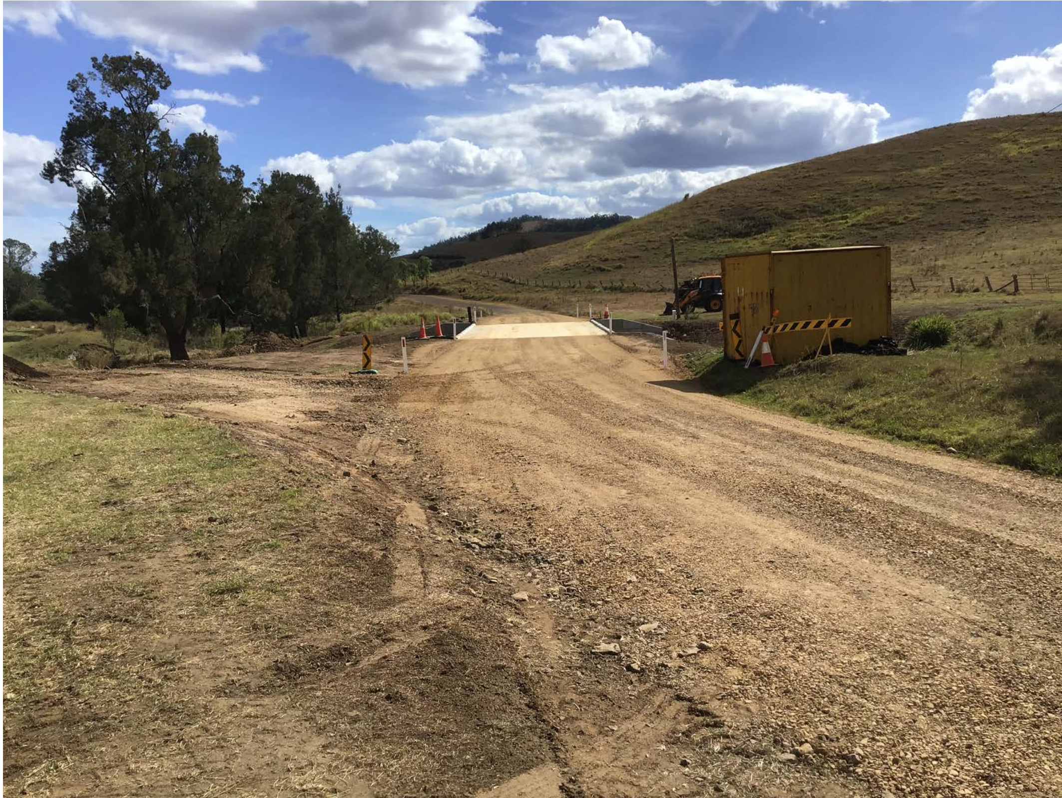
Five Mile Culvert (was bridge) Approaches, now sealed.
