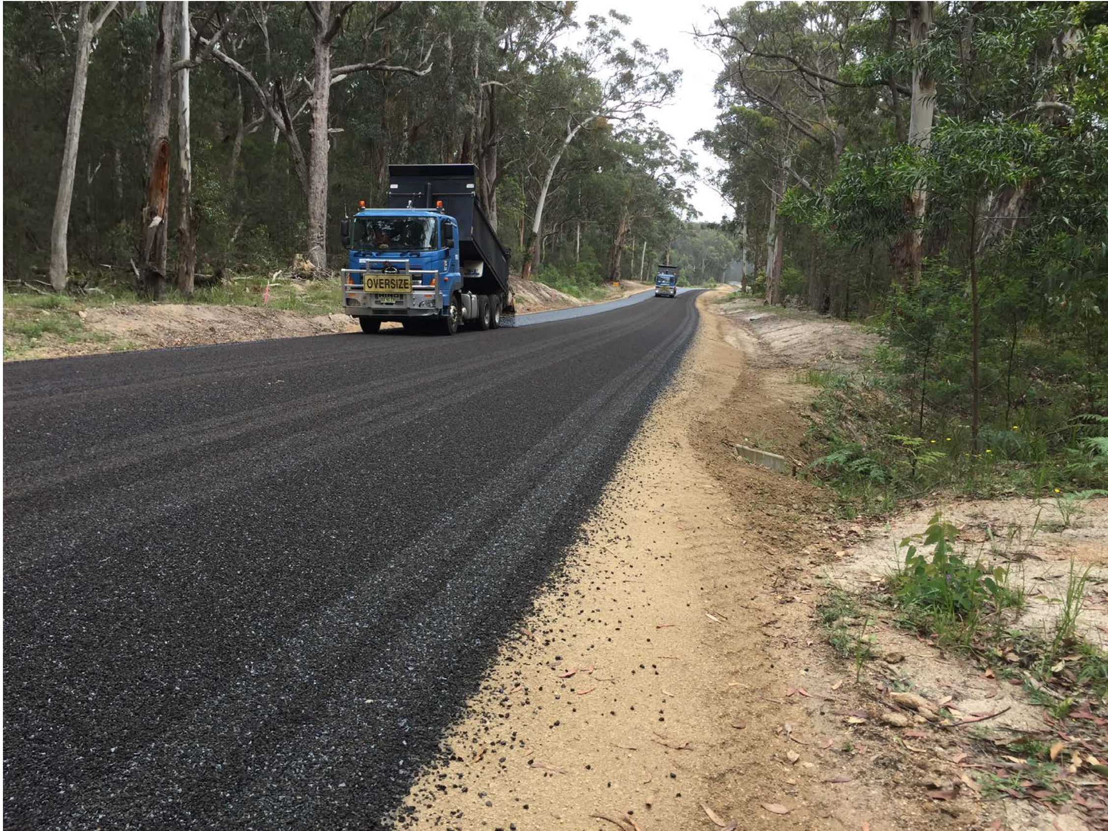
Sealing Bald Rock job.
