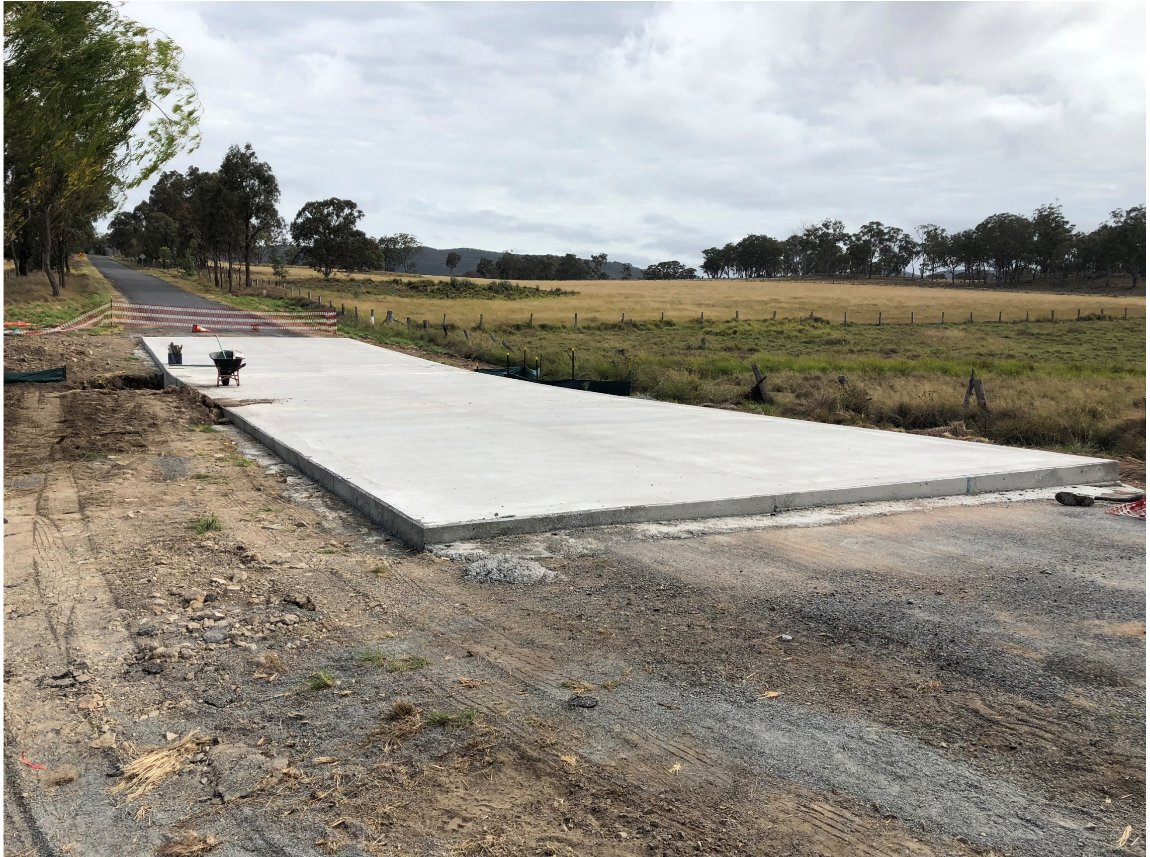
Sunnyside Platform Rd – causeway curing – expect to open 28 th February
