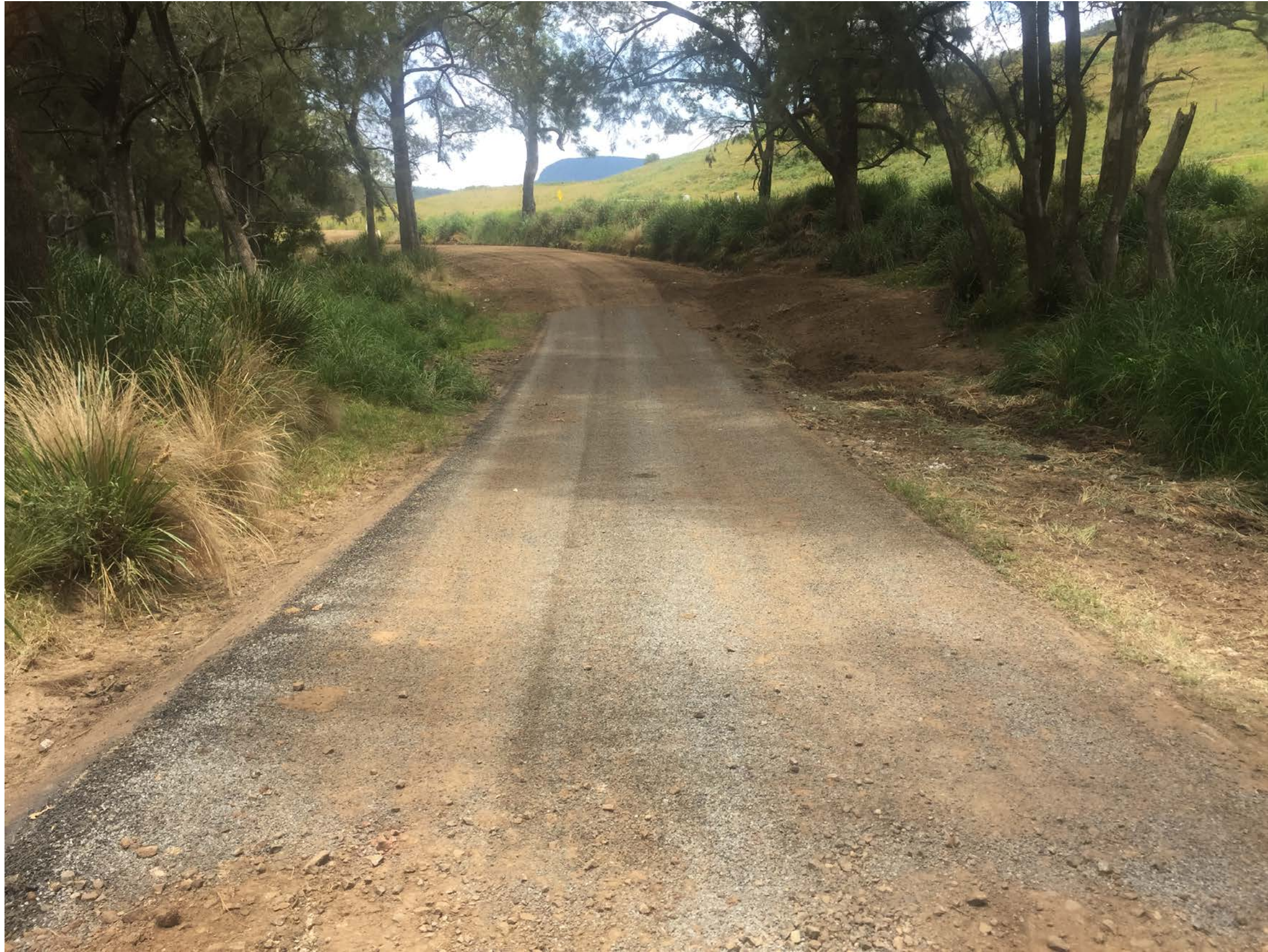
Headgate NDRRA Floodway Repairs
