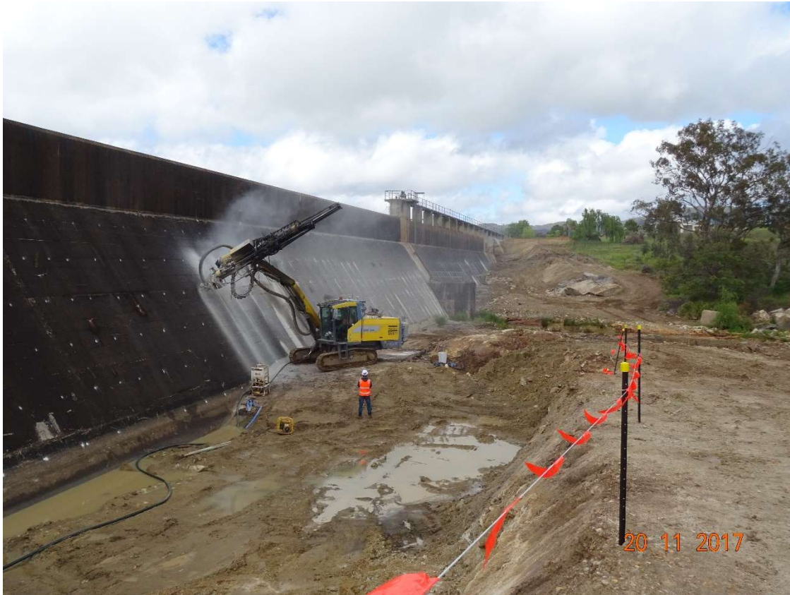
Drilling Anchors RH Abutment
