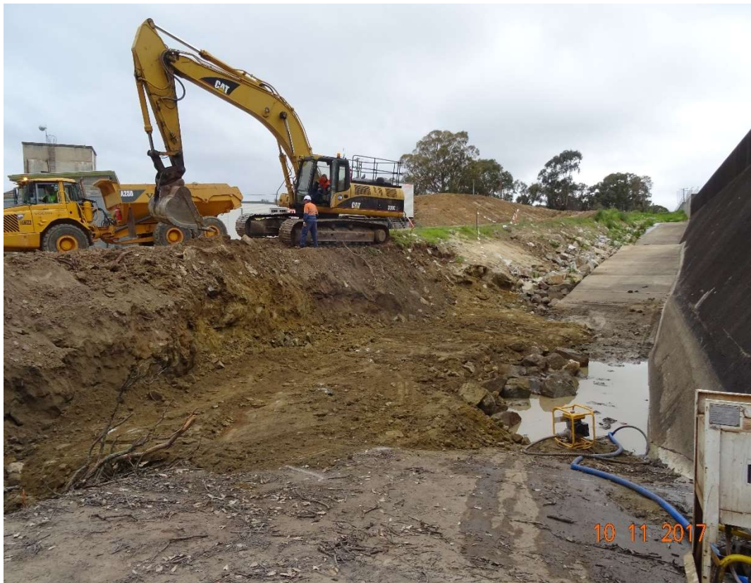
Excavation on RH Abutment
