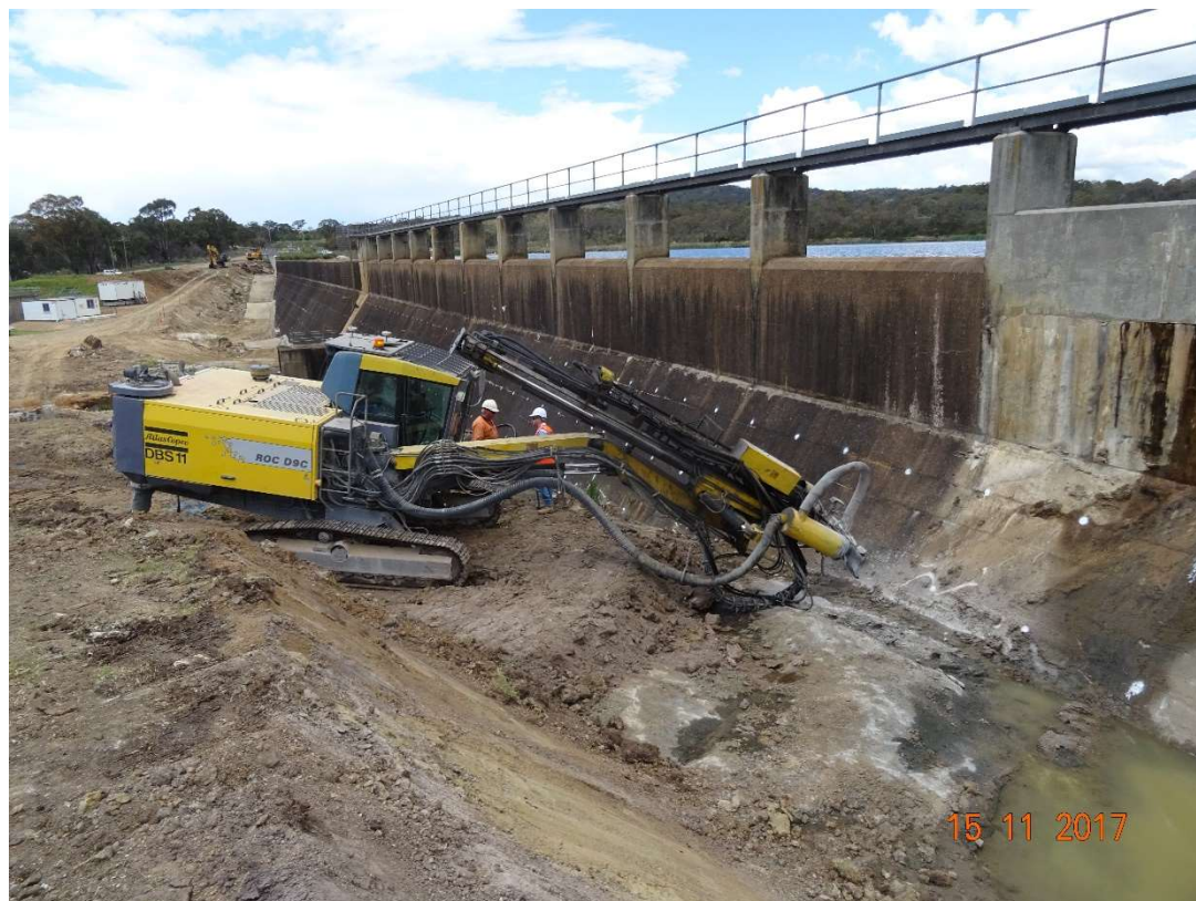
Drilling Upper LH Abutment Anchors
