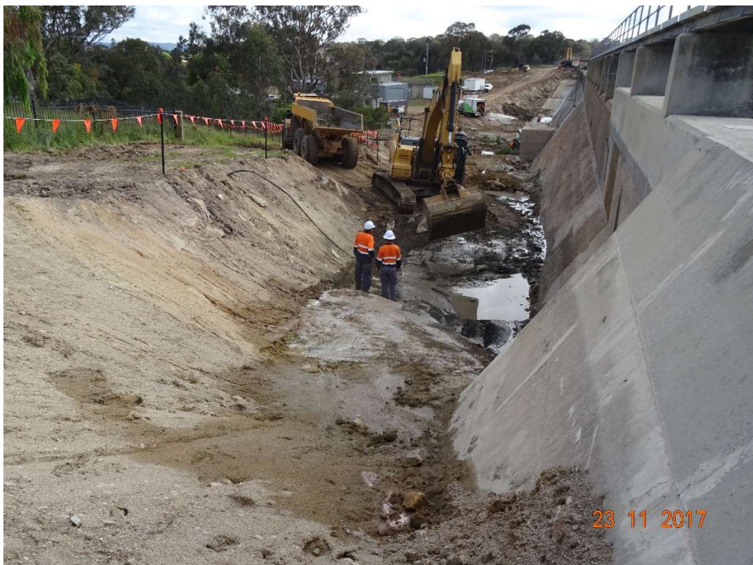
LH Abutment Foundation Clean
