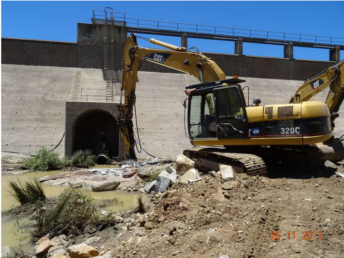
Excavation of Valve House Extension
