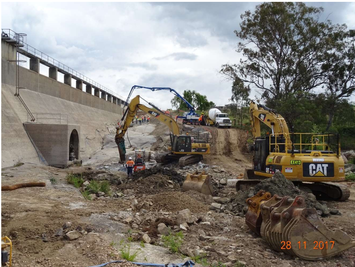
Pouring Dental Concrete LH Abutment
