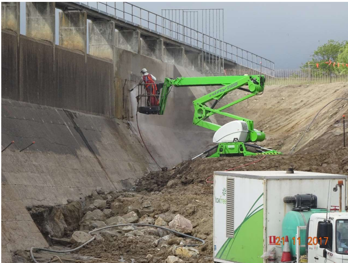
Hydro-Cutting Dam Wall Concrete
