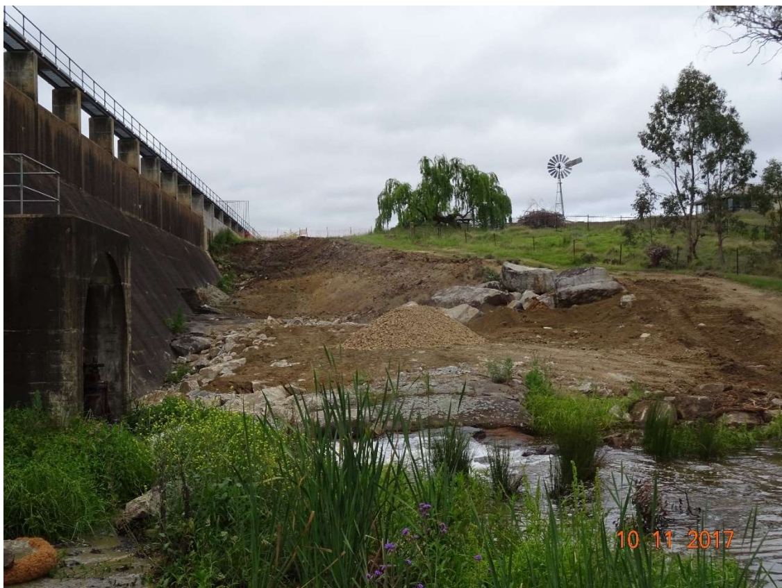
Excavation on LH Abutment
