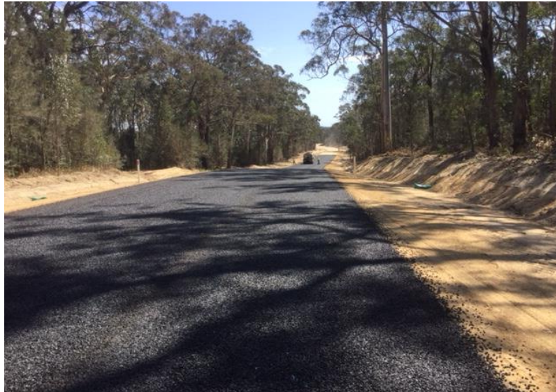
Sealing the 30km to 31.5km section of the Mount Lindesay Road
