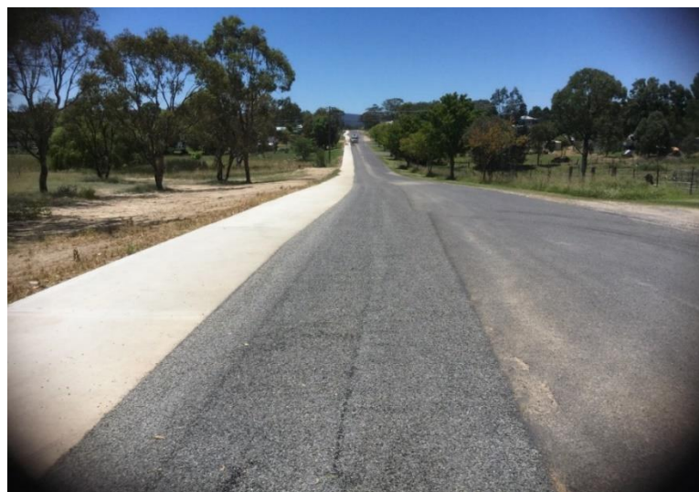
Shared path under construction.
