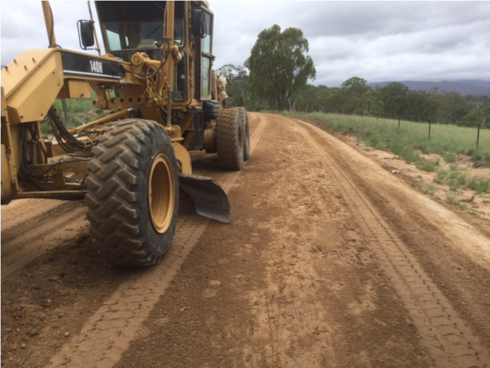
Catching up grading – contract grader grading Sandy Flat Road
