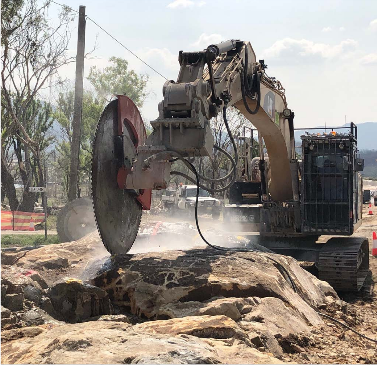
Cutting rock for bore pipeline on Billirimba Road
