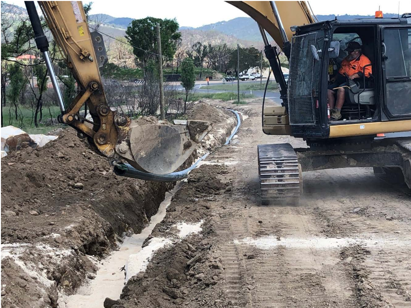
Laying pipe for bores on Billirimba Road
