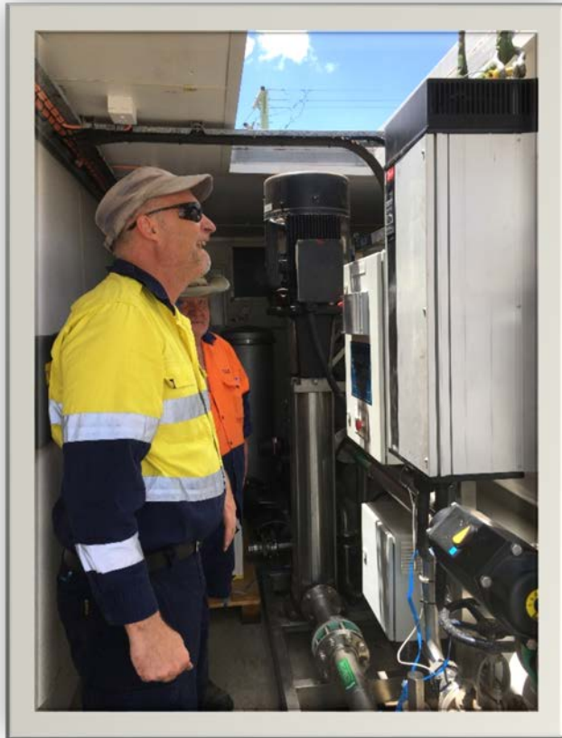
Figure 24,25 ,26, 27,28 & 29 Arrival and installation of new RO system January 2020
